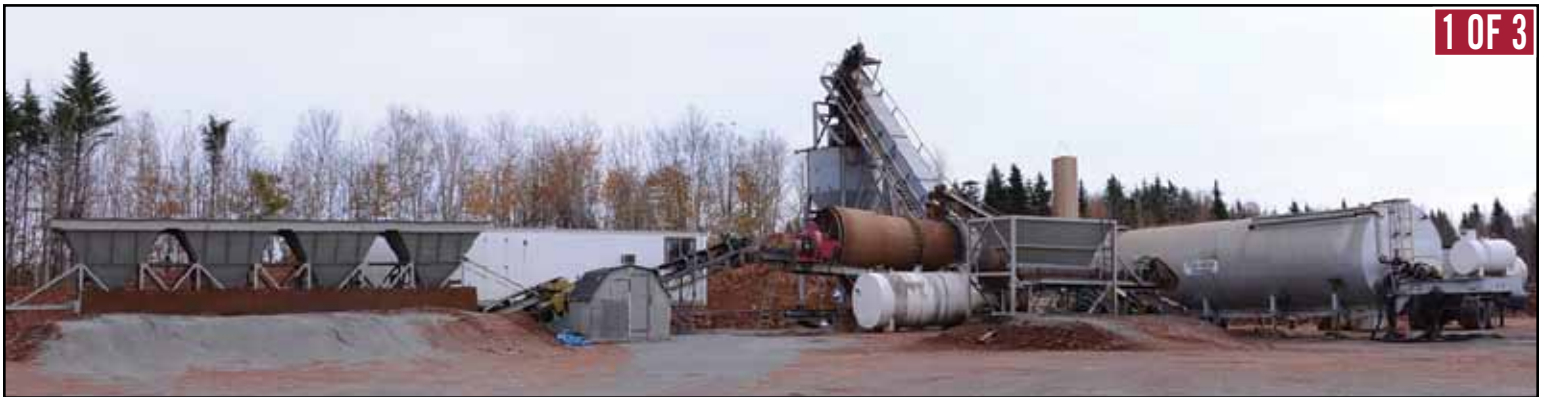
(3) Asphalt Batch Plants
